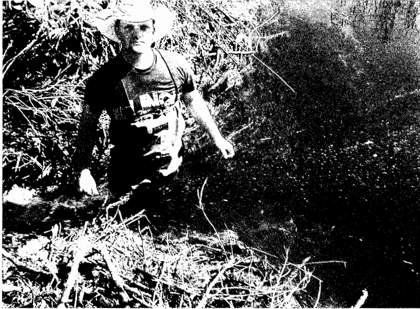
Brad in main dam breach 8/31
