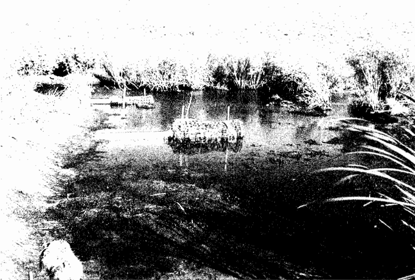
The two Clemson levelers while pond is draining. They used to be completely submerged.
