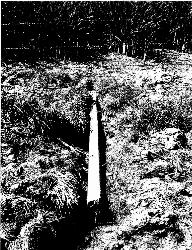
Lateral Pipe drained
